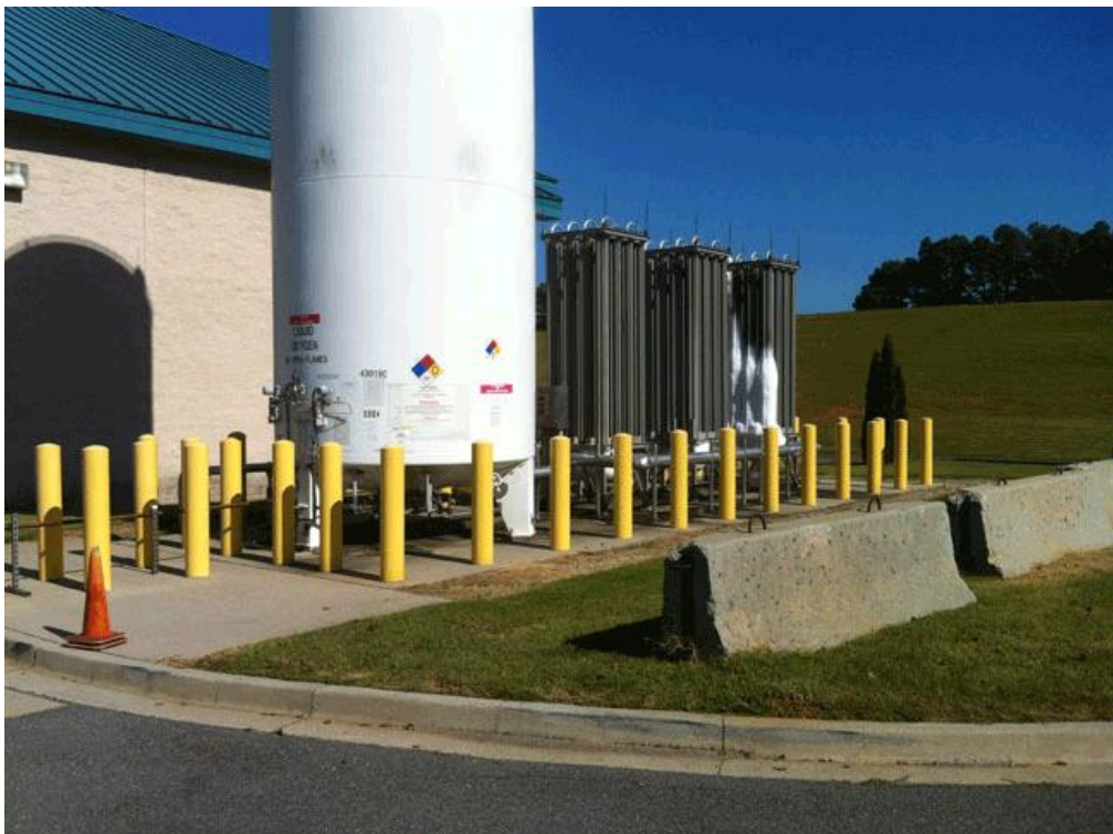
Lanier Filter Plant Liquid Oxygen Tank
