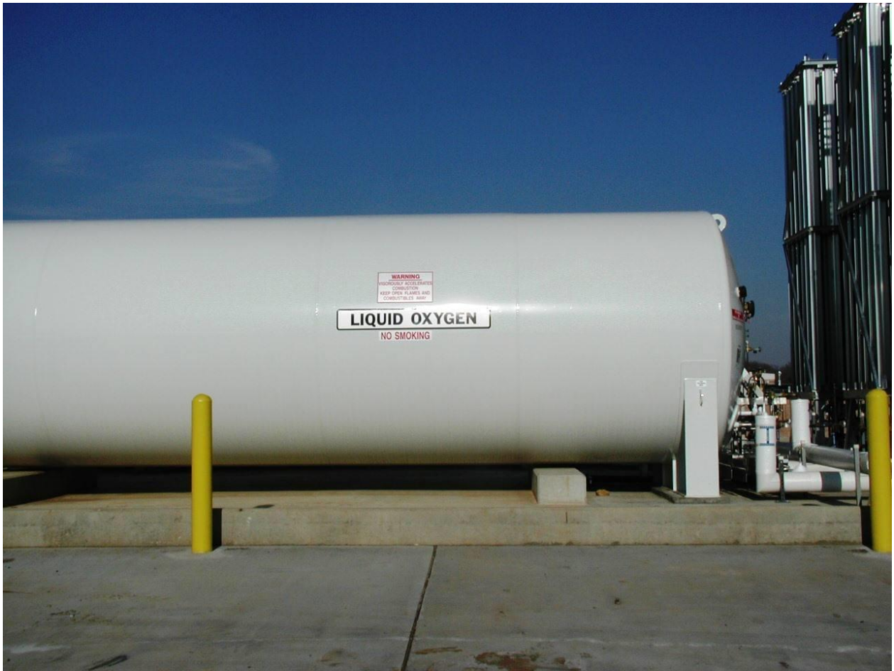
Lanier Filter Plant Liquid Oxygen Tank
