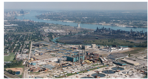
1.7 bgd GLWA WRRF Improvements
