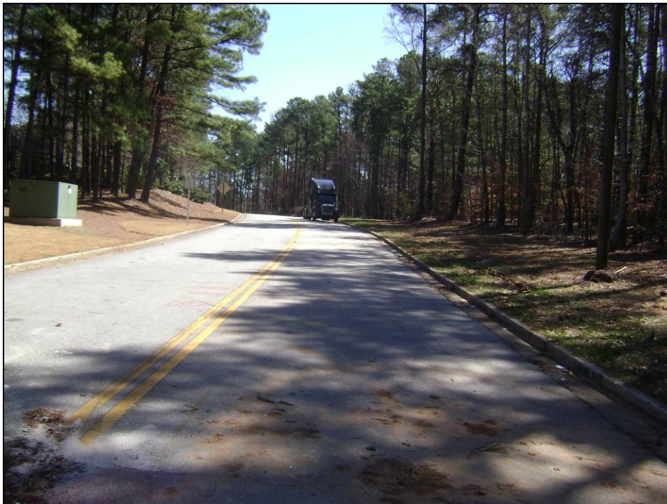
Street scene looking East along Jones Mill Road Subject on Right
