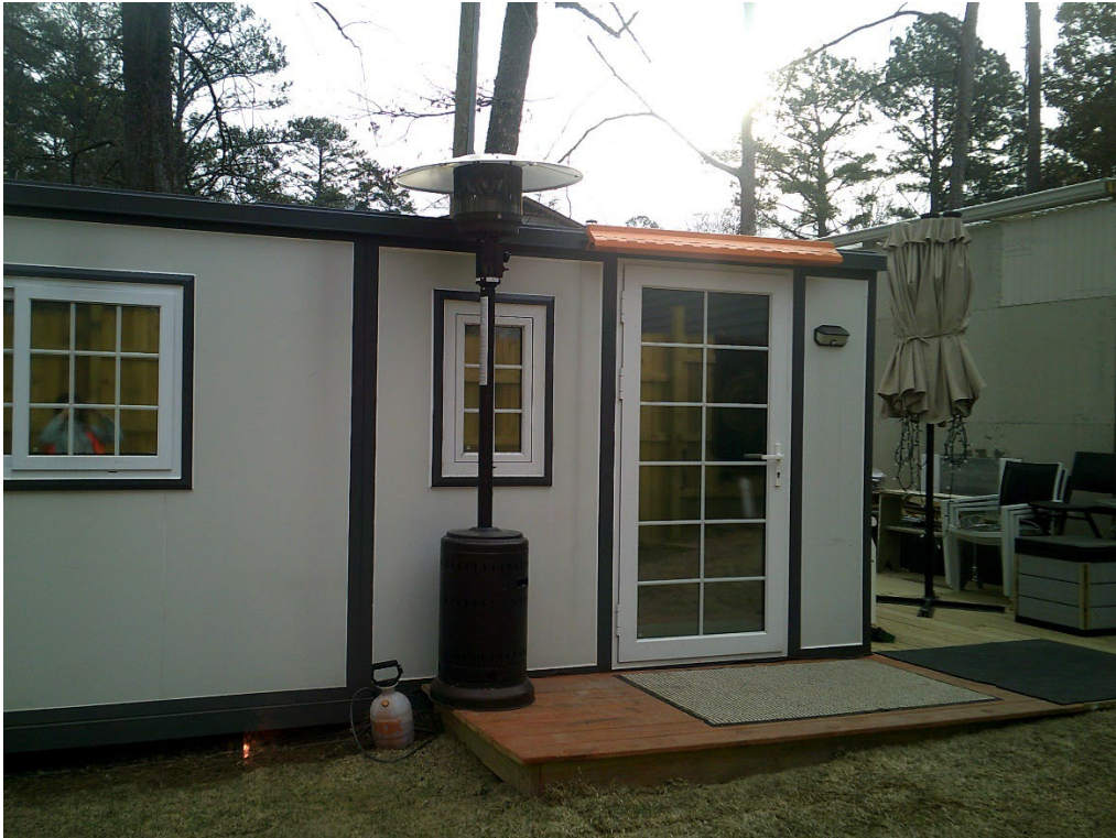
View of accessory structure in yard facing North.
