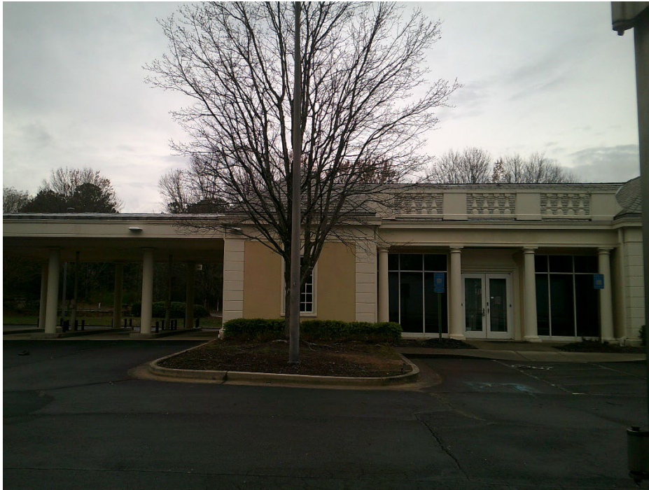
Existing Building (to be demolished)
