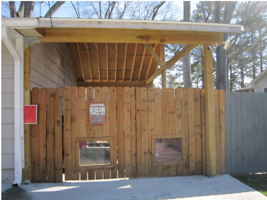
View of carport/roof addition
