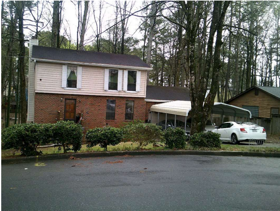
View of the Principal Building
