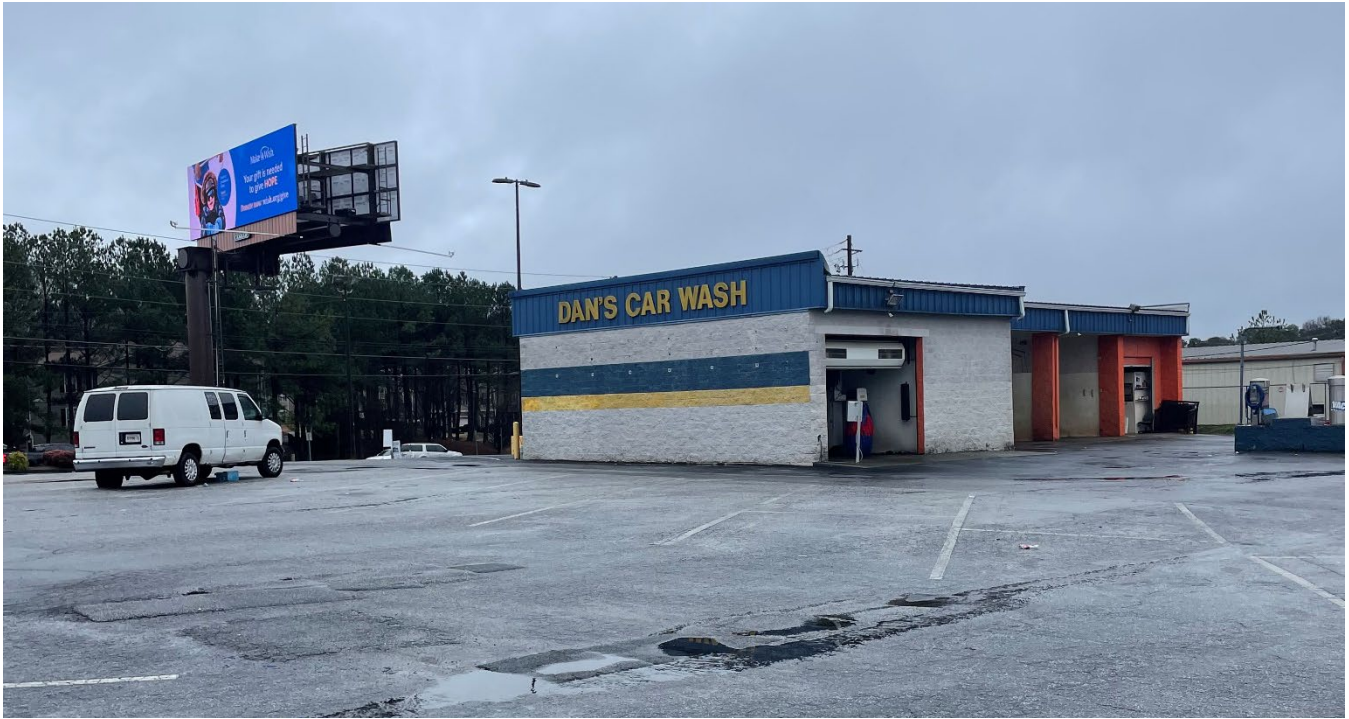
View of the Principal Building
