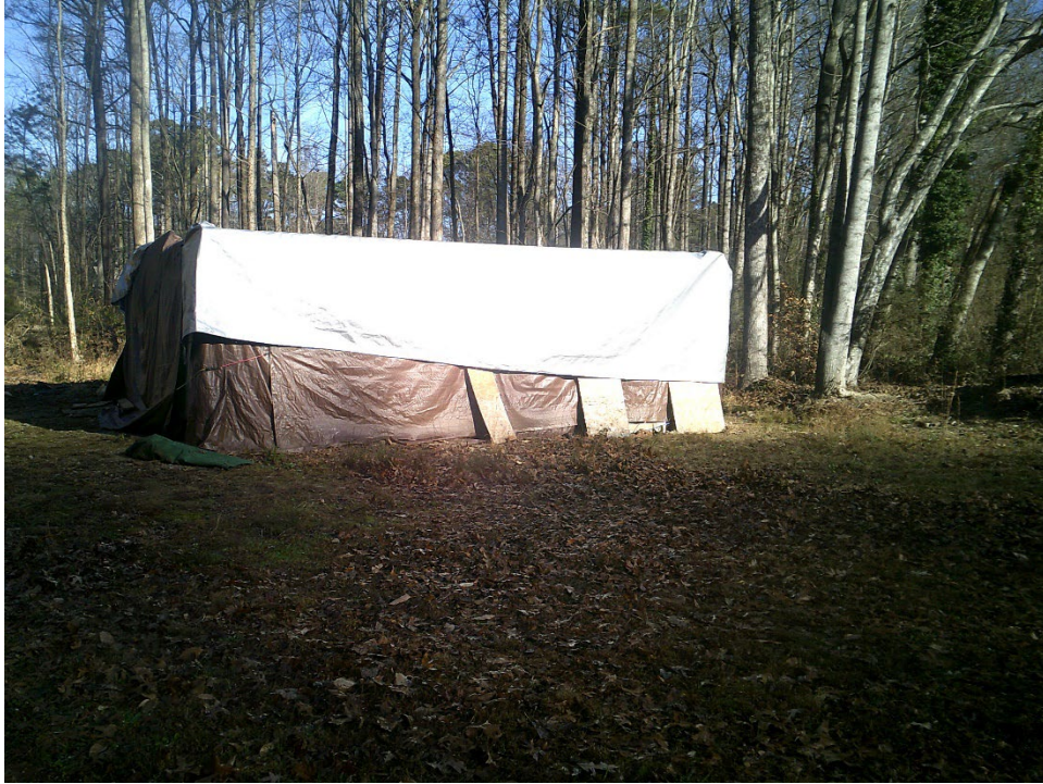
Second view of structure
