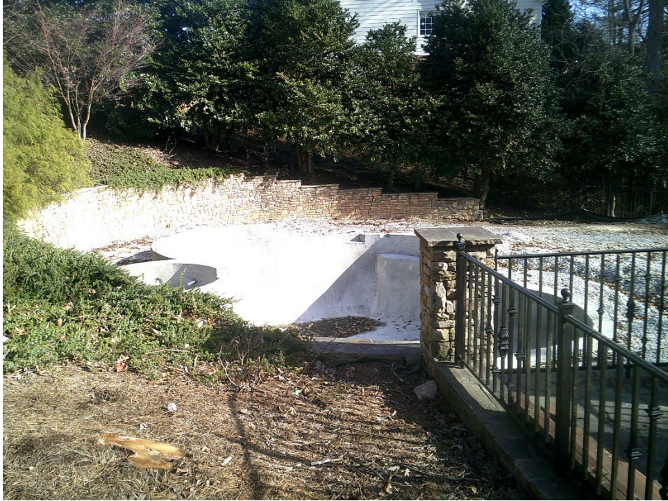
View of accessory structure
