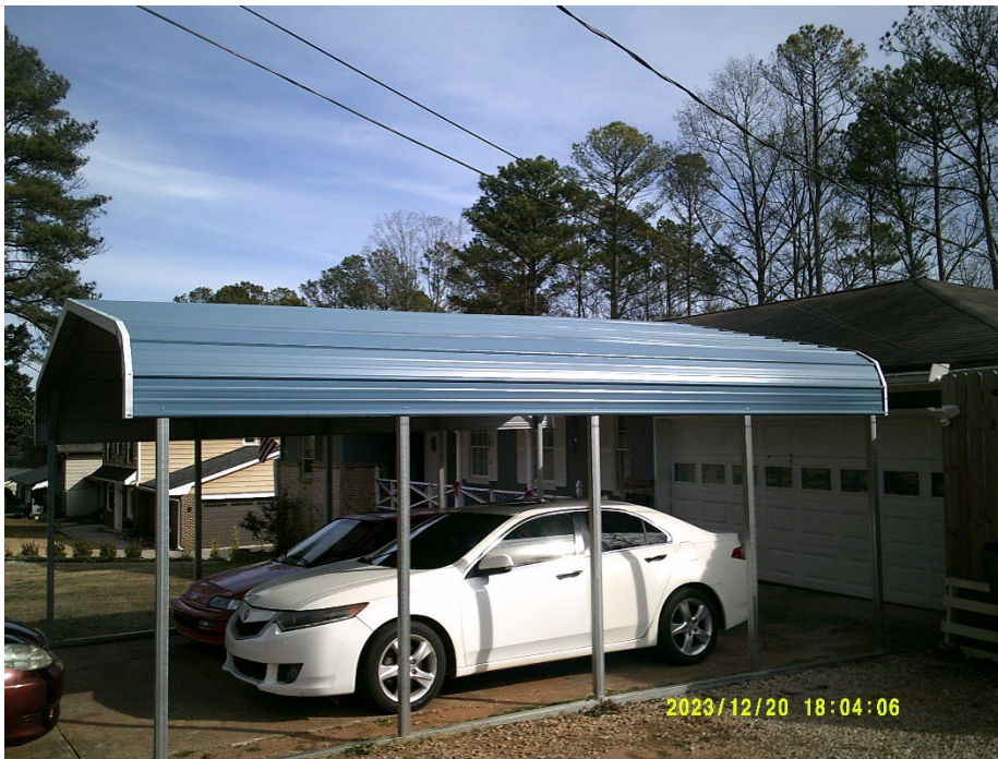
View of the accessory structure
