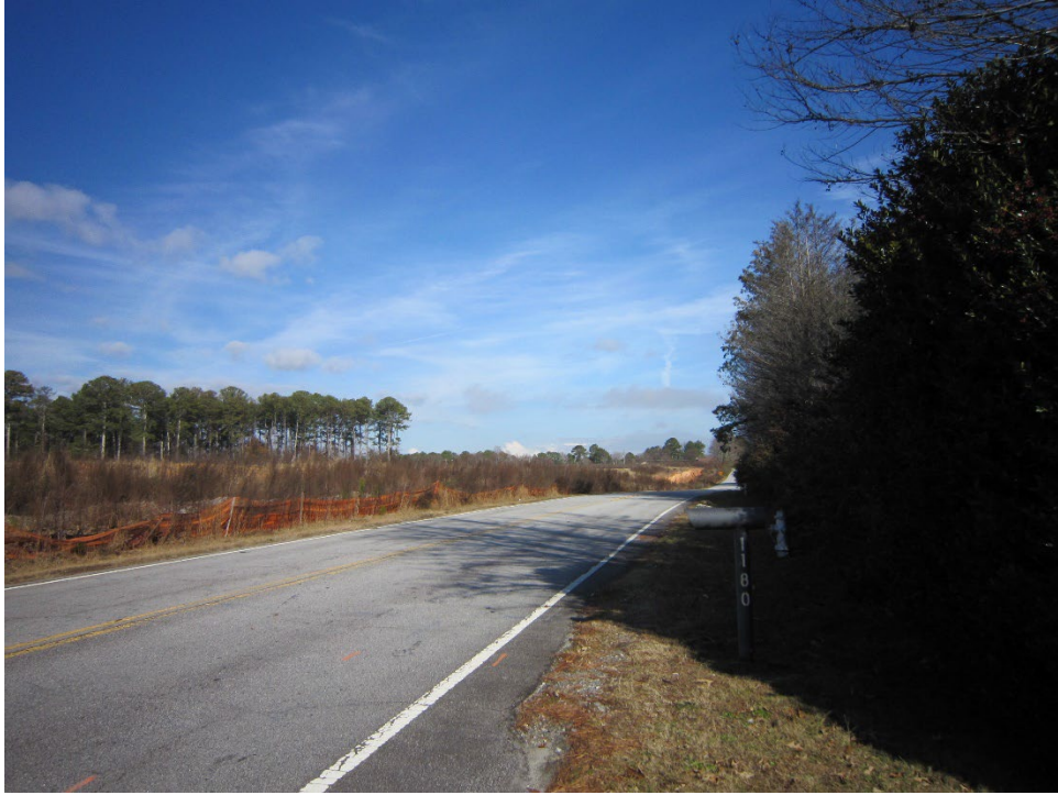
View of right-of-way facing east
