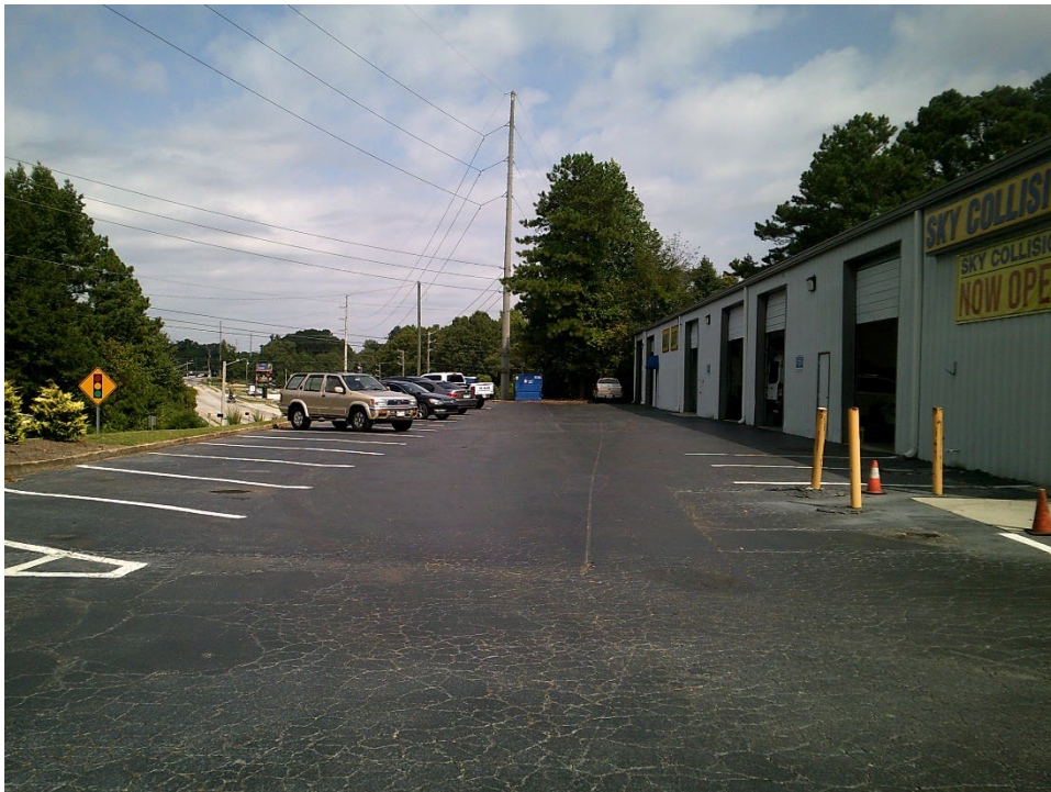
View of the western side of the building with the bay doors and the main parking area
