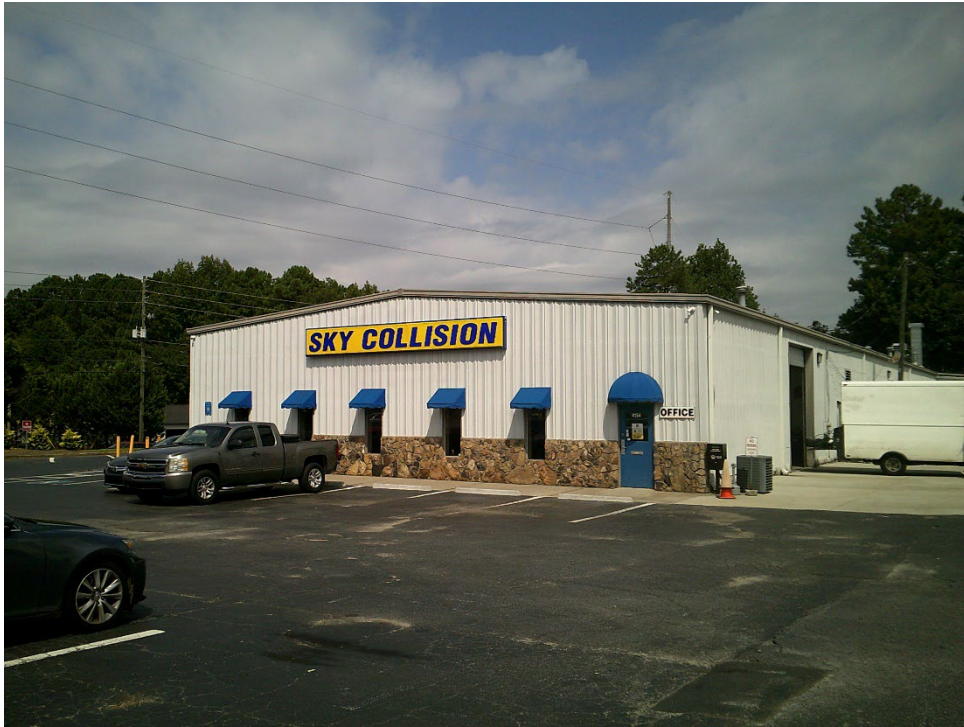
View of the front of the building
