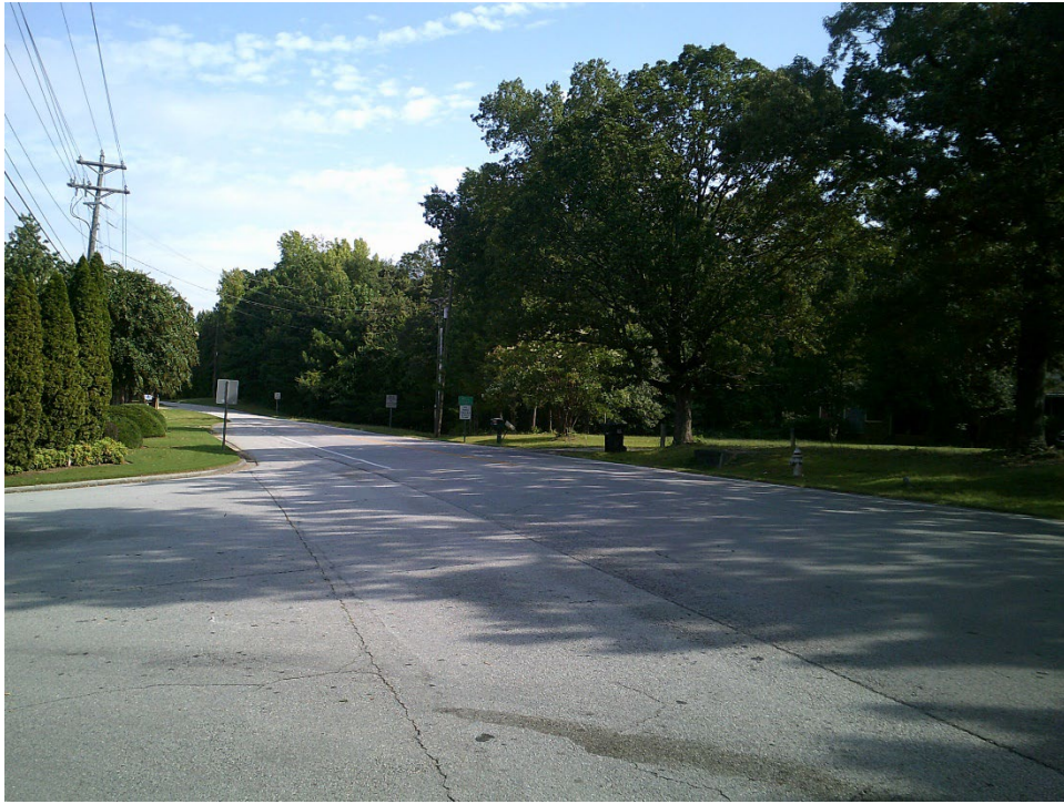
View of north bound Ridge Road
