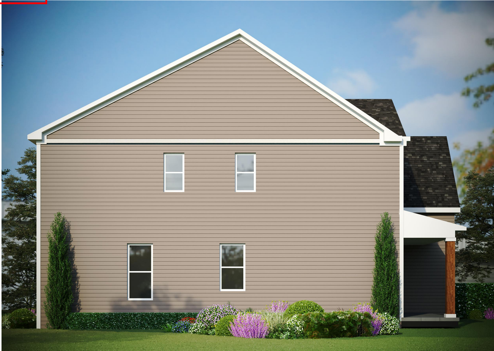
FIBER CEMENT LAP SIDING
