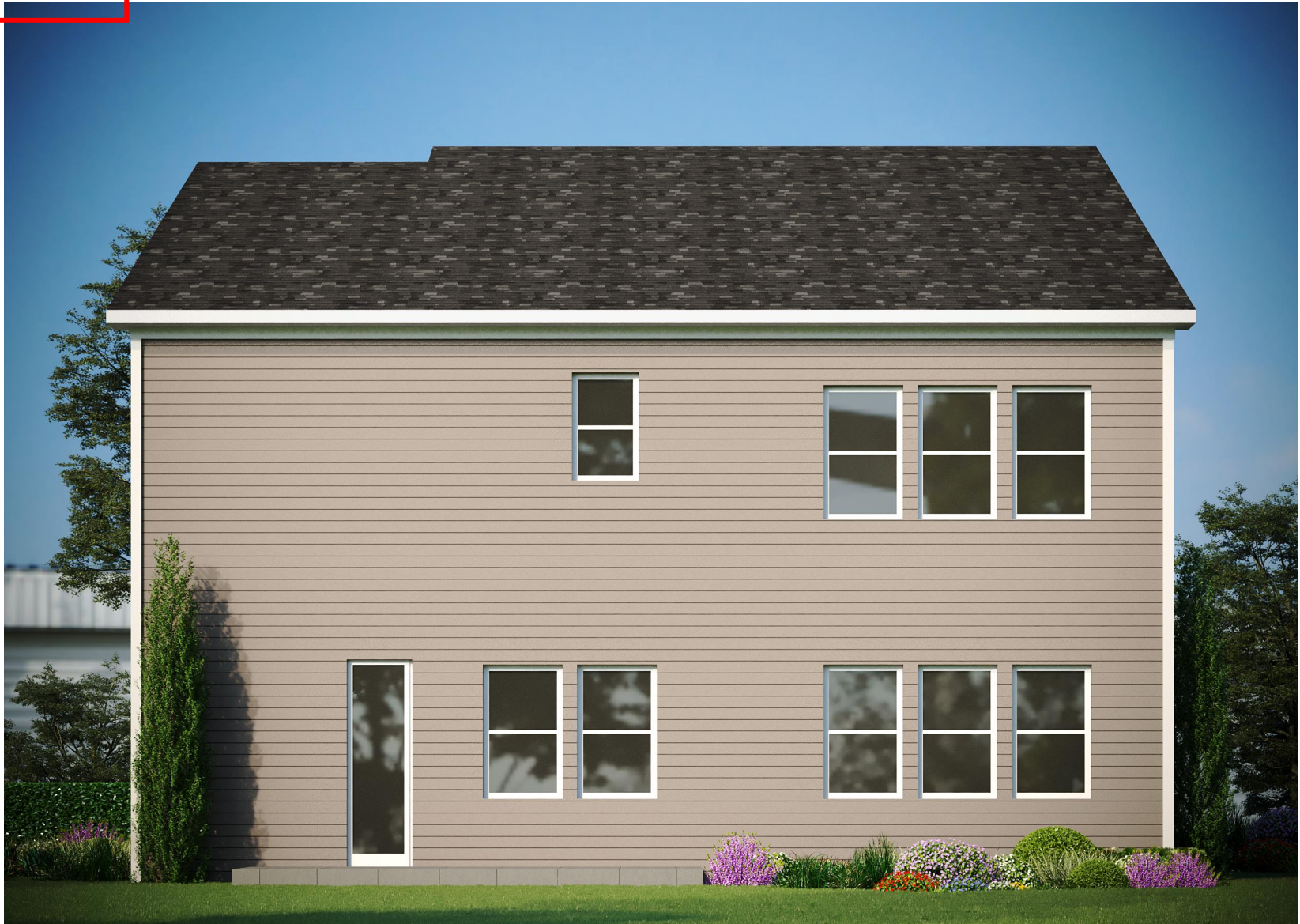
FIBER CEMENT LAP SIDING
