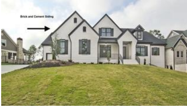
Front – brick and cement siding
