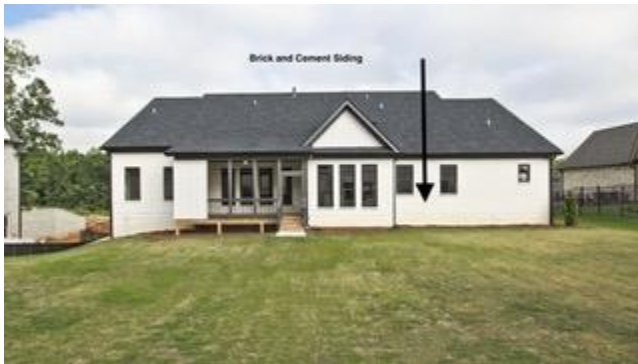
Rear – brick and cement siding
