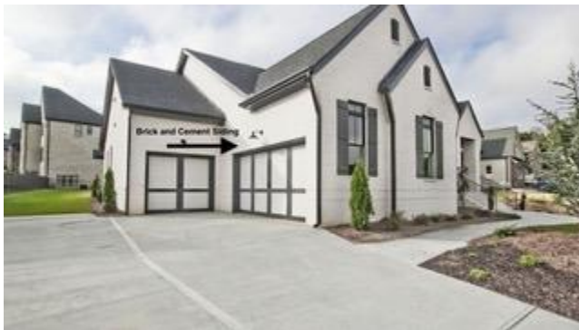
Side 1 – brick and cement siding
