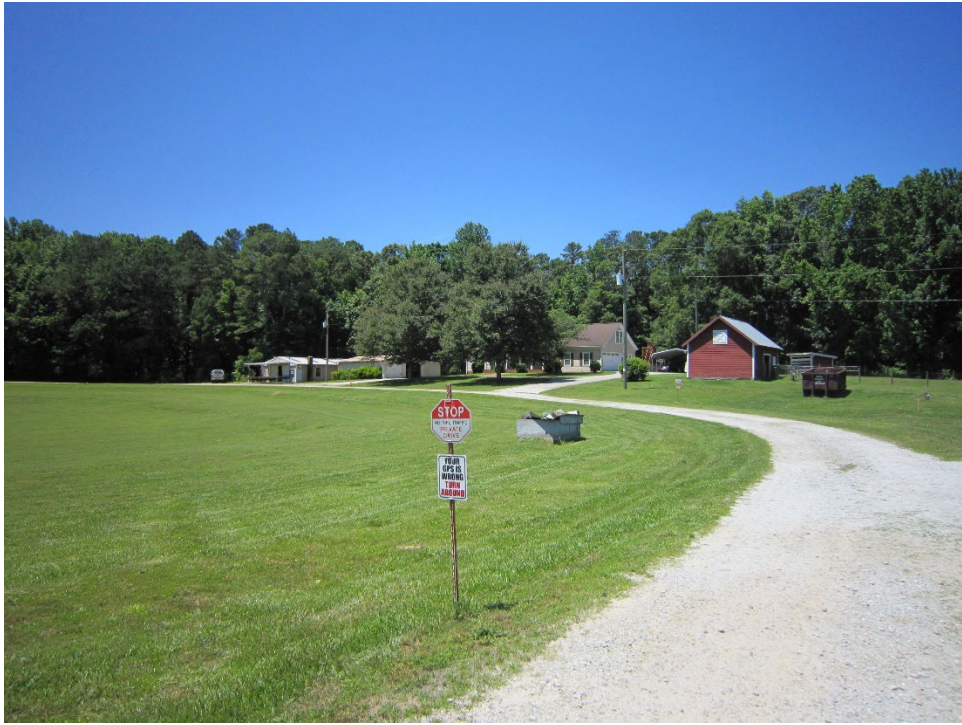
View of existing structures
