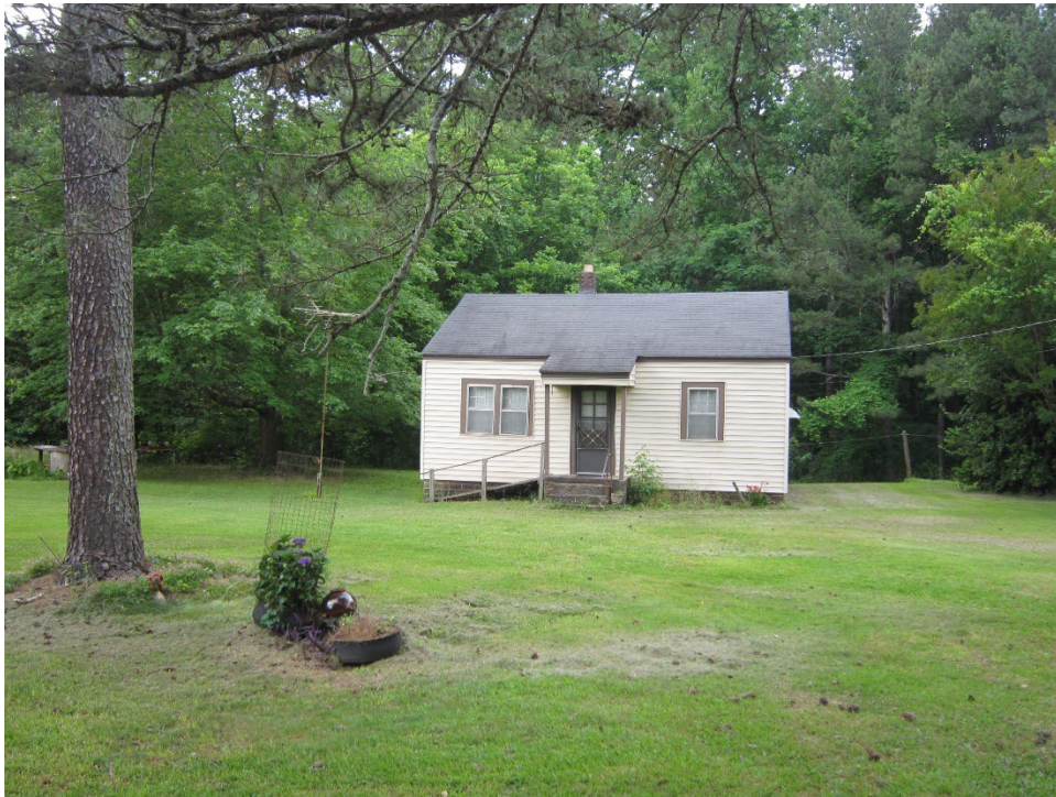
View of existing residence on the site
