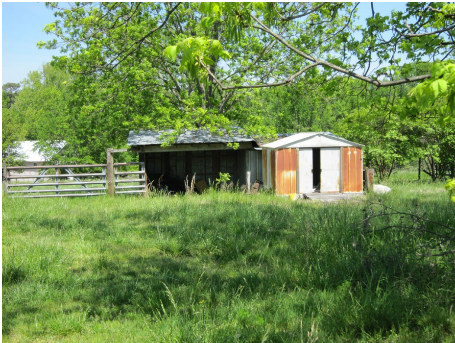
View of metal shed structure
