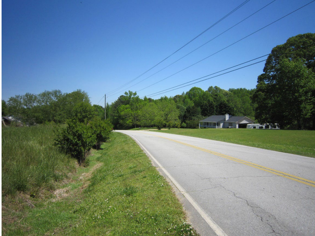
View facing north along Clack Road
