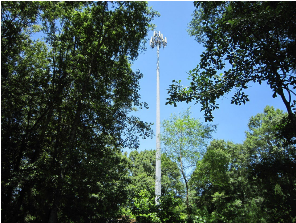
View of monopole to the south
