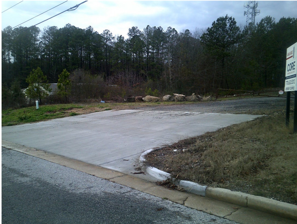
View of existing entrance to property
