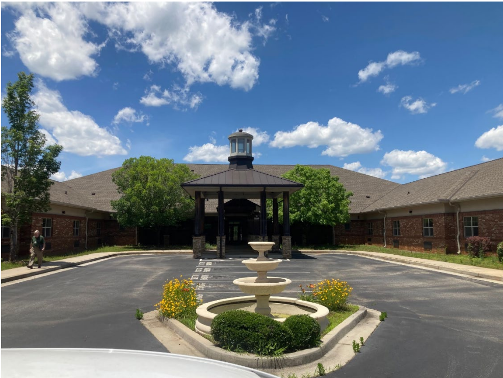
View of the front entrance of the facility
