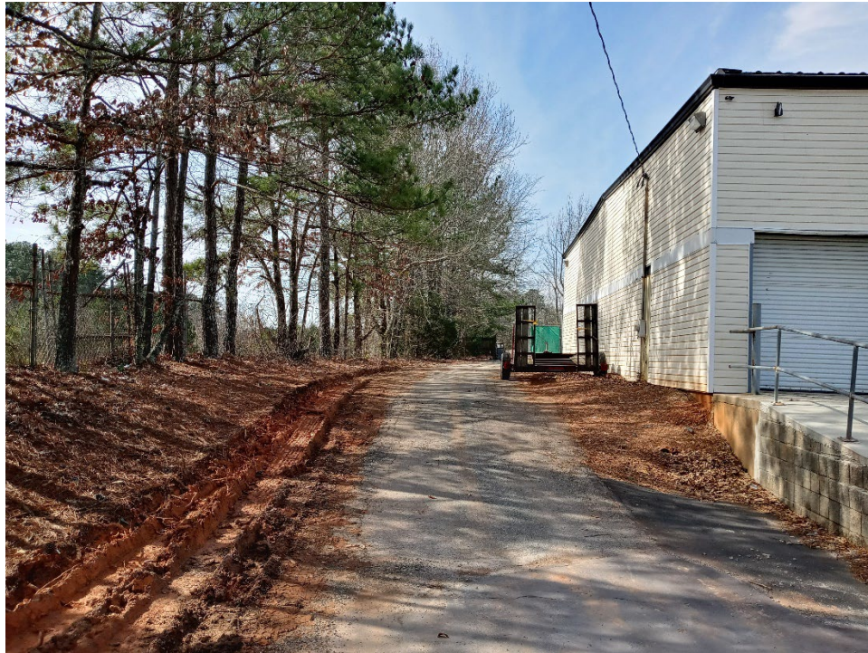
Southern property line where buffer reduction is being requested
