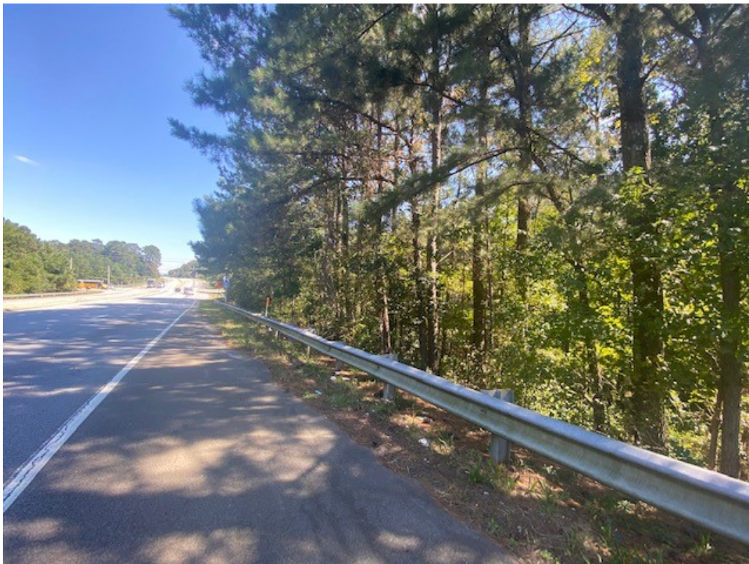
Frontage along Lawrenceville Highway
