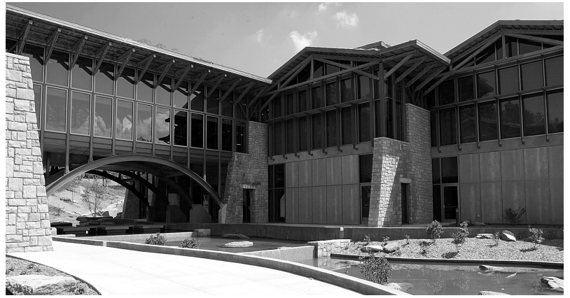
The Gwinnett Environmental & Heritage Center is a living laboratory of environmentally-sensitive construction methods and materials.
