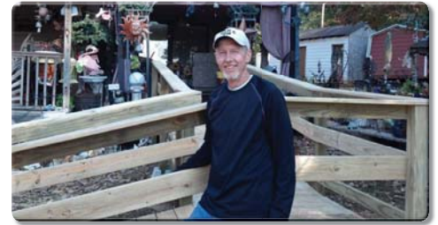
Harvey Anderson surveys completed access ramp
