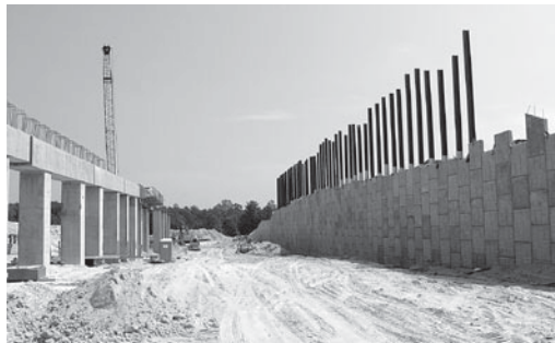
Sugarloaf Parkway Extension Construction
